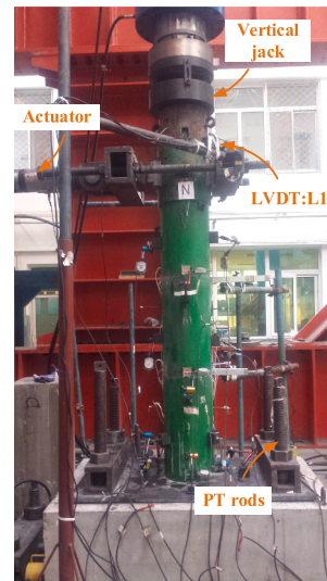
(b) picture of PS-CFST under test
